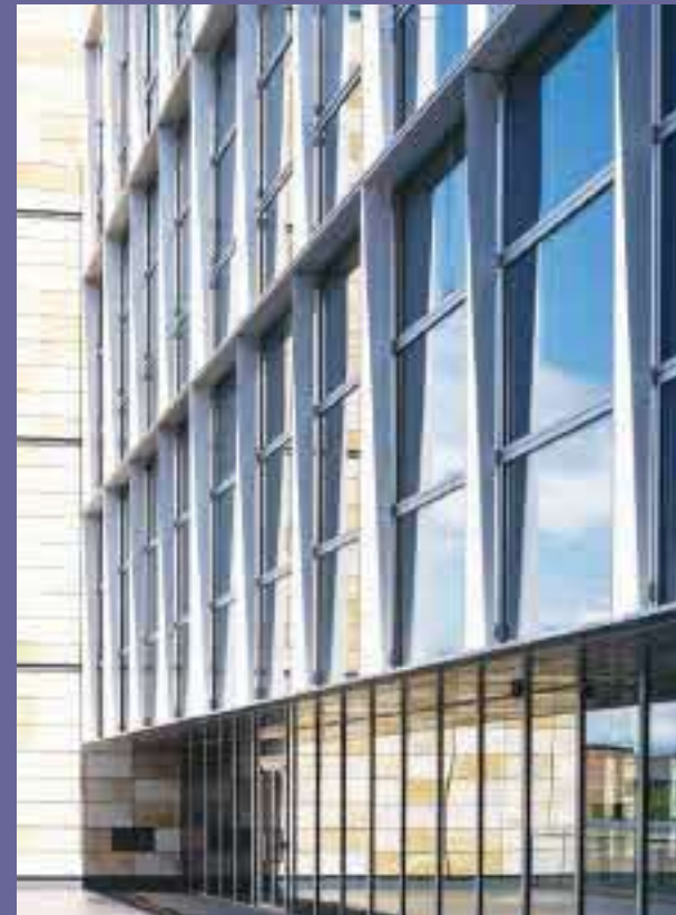
Old windows at One Triton Square were removed, repaired and refitted. Photo courtesy of Arup
