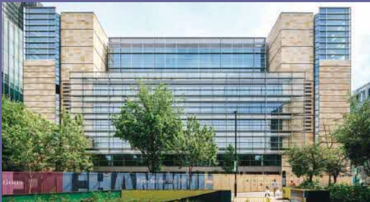
One Triton Square was renewed through a deep retrofit. Photo courtesy of Arup
