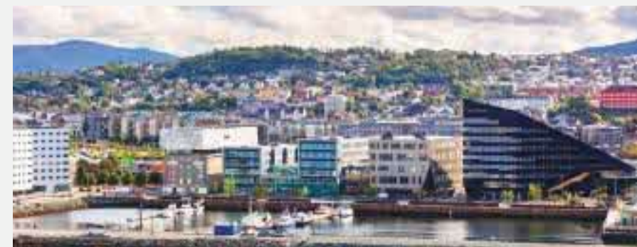
Powerhouse Brattørkaia supplies surplus energy to its surrounding neighbourhood.
