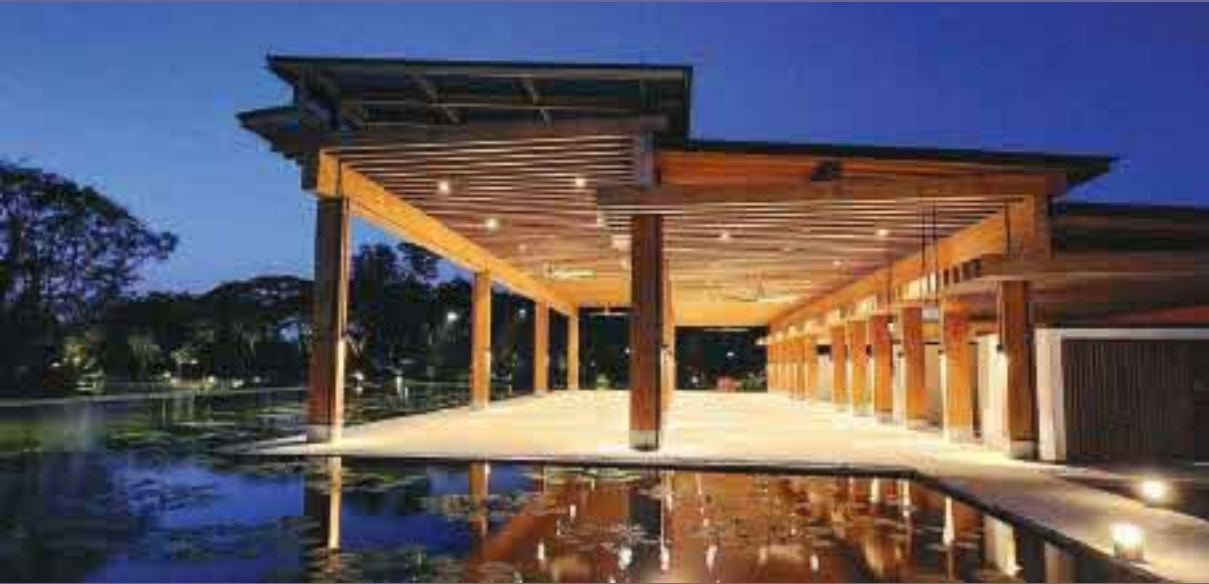
At Jurong Lake Garden's Japanese Garden, advanced Mass Engineered Timber was used as a sustainable innovation for construction of the Water Lily Pavilion (above) and the Guesthouse (left). Photos courtesy of National Parks Board
