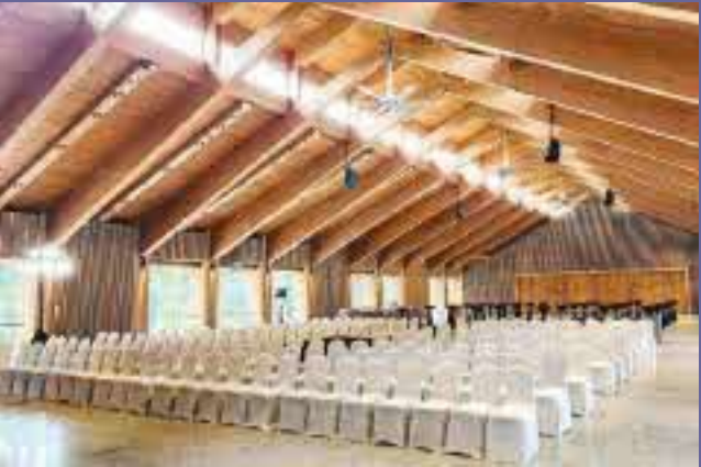
At Jurong Lake Garden's Japanese Garden, advanced Mass Engineered Timber was used as a sustainable innovation for construction of the Water Lily Pavilion (above) and the Guesthouse (left). Photos courtesy of National Parks Board
