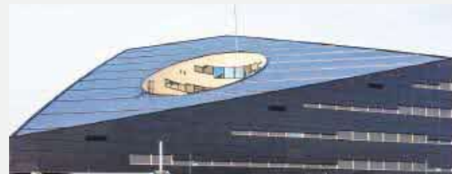
The roof of Powerhouse Brattørkaia is clad in solar panels.
